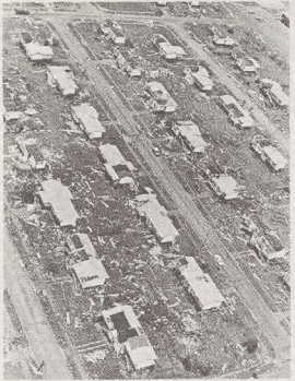
Previously comfortable married accommodation for families on Base, but after Cyclone Tracy struck, the married path became a shambles. As RAAF News pik shows, a few of the married quarters managed to retain some roofing, but all were substantially damaged in the "Big Blow" to add to the heartbreak of Christmas Eve, 1974.
